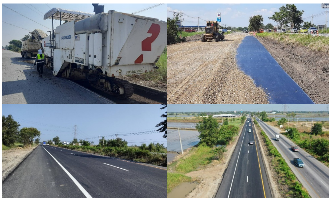
Figure 7 Rehabilitation process and project completion.
