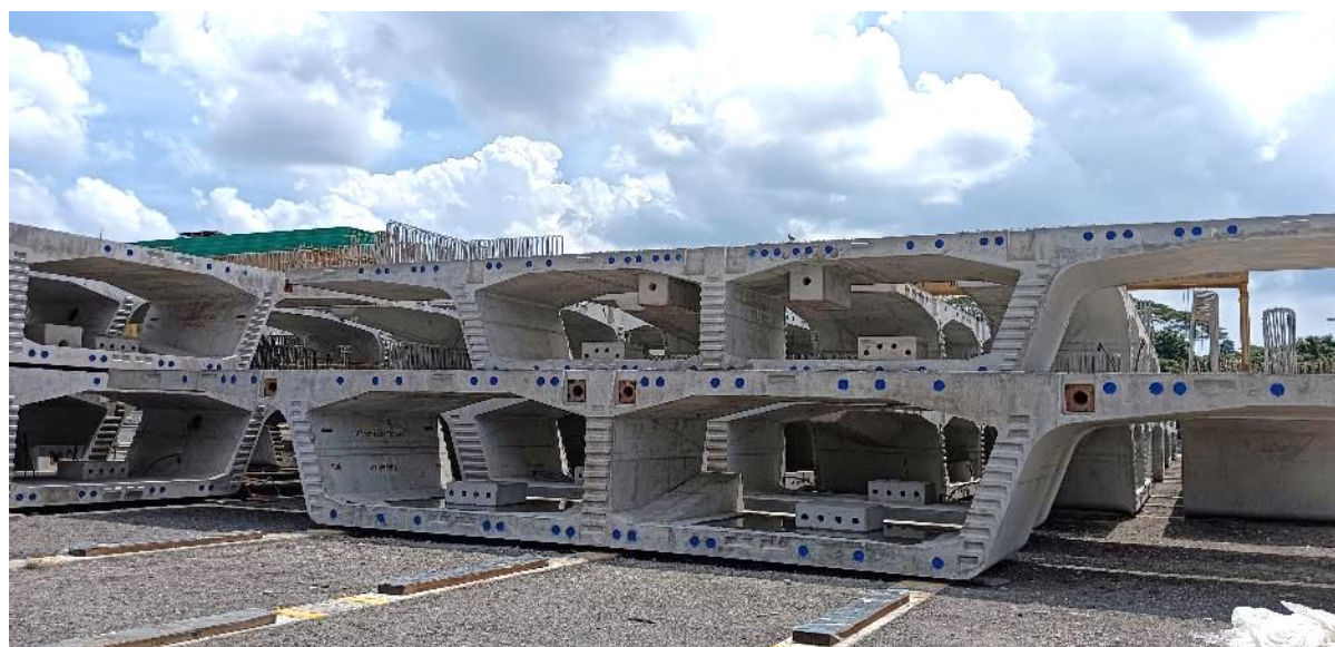
Figure 5b Picture of casted segments in satisfactory condition.
