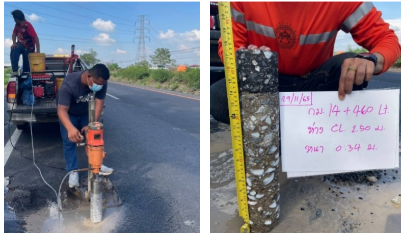
Figure 8 Extraction of a 100 mm diameter core.
