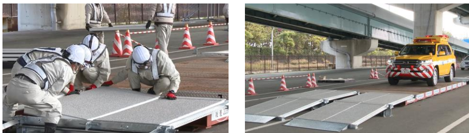
Figure 8 Installation of Bridging Boards Over Bump to Enable Smooth Vehicle Passage.
