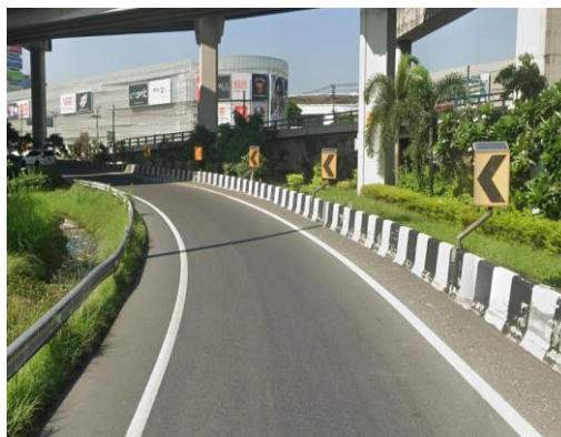
Figure 5 : Using SMA at Motorway#9's Ramp by DOH
