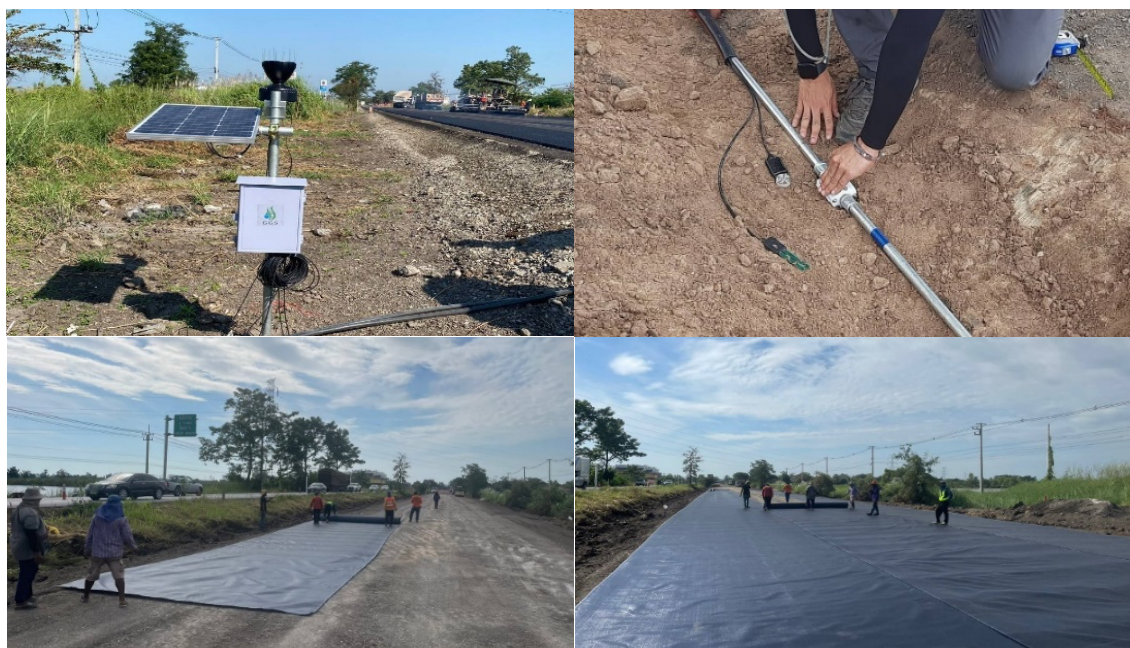
Figure 6 Installation of field monitoring instrument and IPED geotextile.
