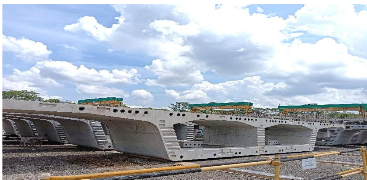
Figure 5a Picture of casted segment in satisfactory condition.
